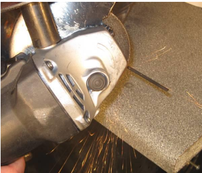
Cut the innercore at the mark
