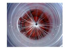
By cleaning of round ducts you can choose either to rotate left or right
